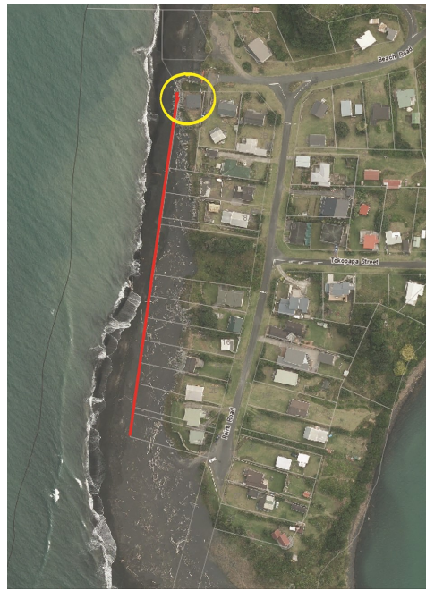
Photo: A 2012 photo shows the effect of the coastal erosion as it encroaches 4 metres inland posing a real danger to the Point Rd properties. The property shown in the circle was removed following significant erosion events in 2013.
